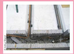
Floor beams are cast onto polystyrene panels and the reinforcement is tied into the concrete core.
