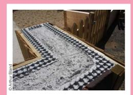
Concrete is poured into the insulating formwork in 0.5 m high 'ribbons' on a continuous basis up to 3 m.
