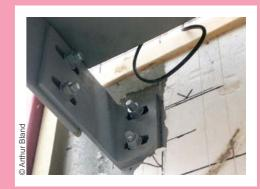
Metal fixings are cast into the concrete core. Care must be taken to replace insulation where it has been cut out.
